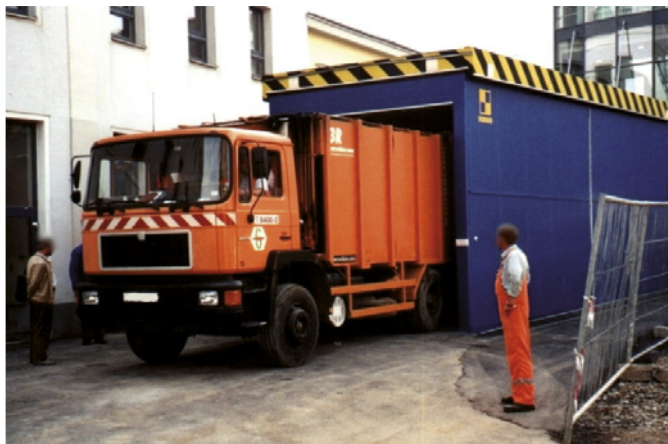
Lorry lifter, platform size: 11.0 m x 3.8 m, Capacity 16 t
